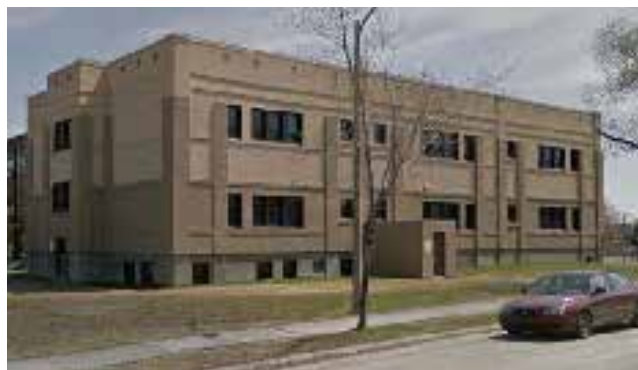
50, avenue Murdoch (école Notre-Dame-de-Protection). Google Street View, 2013.
